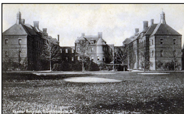
1902 After the renovation
