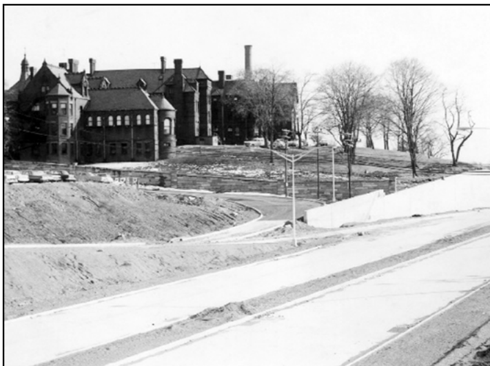
Construction of Route 9
