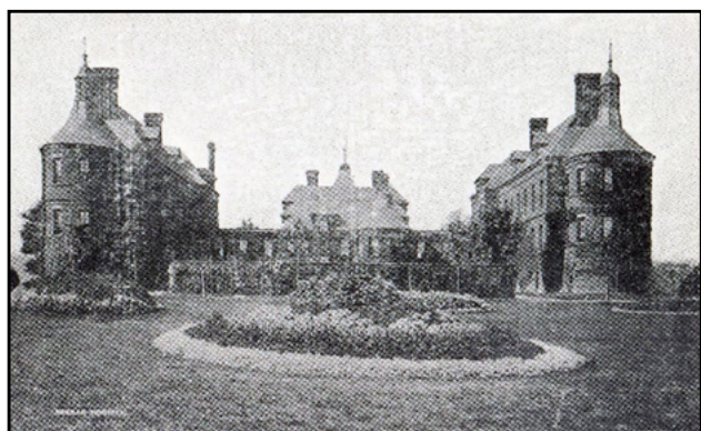
1900 Before the renovation
